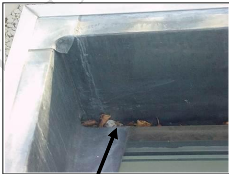
Close up of small box gutter
