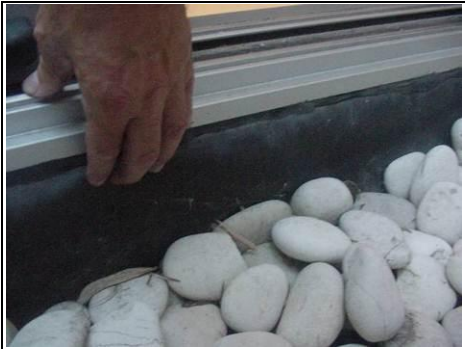
Mono-ply used on rear light well
