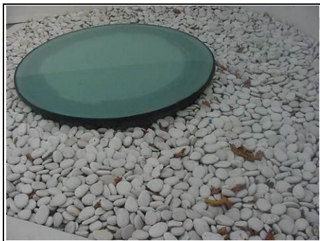
Roof window into the front bedroom below
