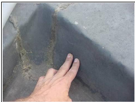
Checking the detailing
