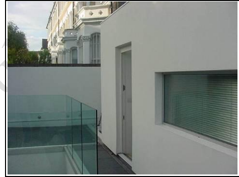
Front elevation right view
