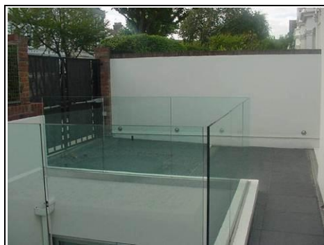
Front parking area
