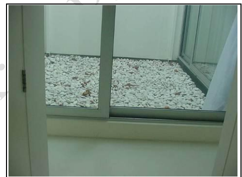
Front light well/patio-bottom
