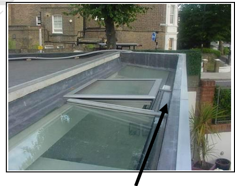
Roof windows above the kitchen with small box gutter
