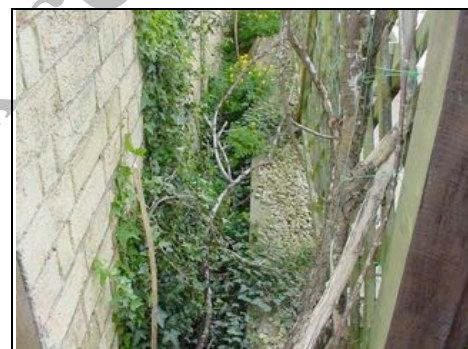
Vegetation to right side area
