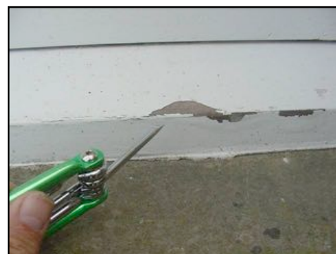
Flaking paint to timber windows
