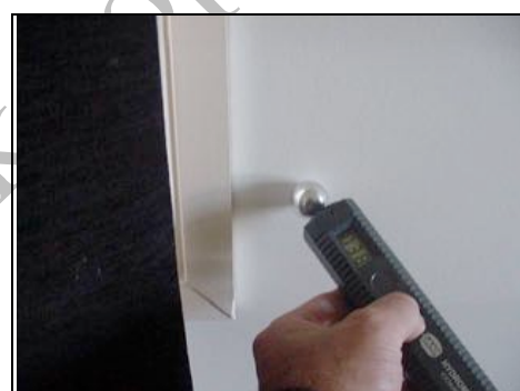
Testing for lateral dampness
