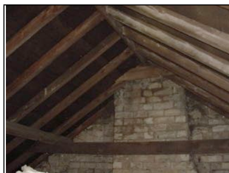
General view of inside of roof
