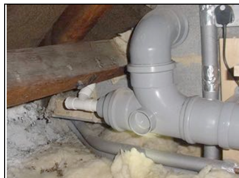
Soil and vent pipe within roof
