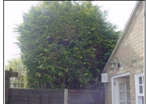
The tree is located in next doors garden but is right next to your property
