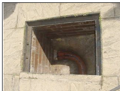
Rear left hand manhole
