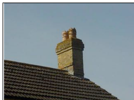
Right hand chimney
