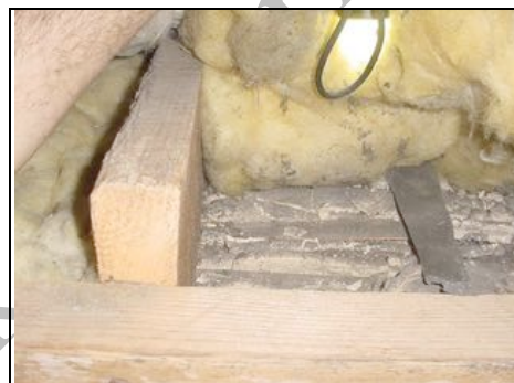
Lath and plaster
