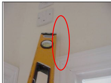
Hairline cracking
