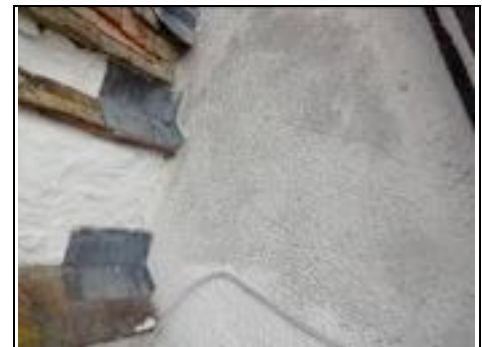
Mastic on lead to right gable
