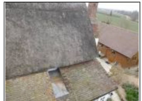
Displaced tiles and in need of repair
