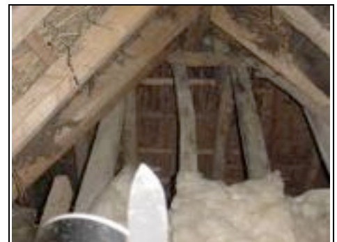
Deterioration/twisting to timbers in left roof
