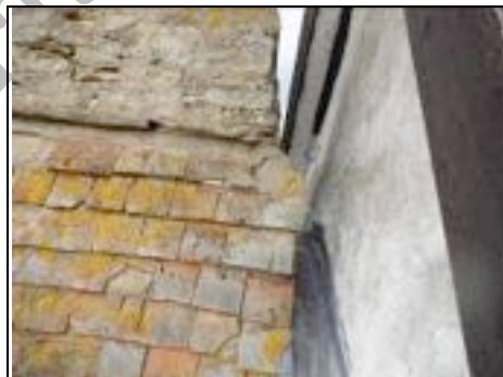
Gap between chimney and main building
