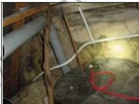
Soil and vent pipe
