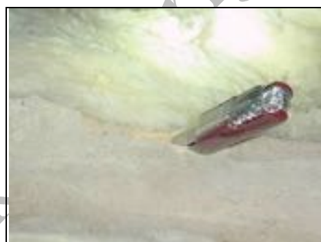
Knife going completely into timber common rafter
