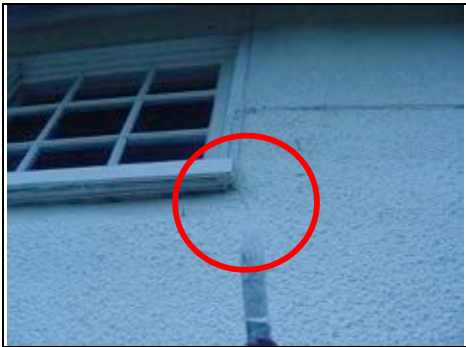
Cracking to the window
