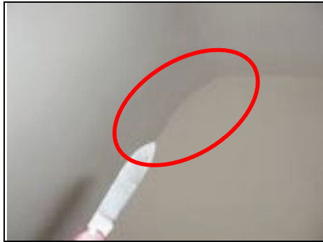
Hairline cracking in master bedroom
