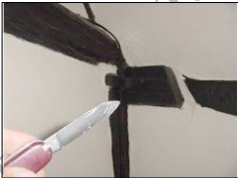
Infill panel with metal brace
