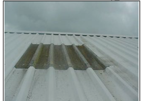
Roof windows in poor condition
