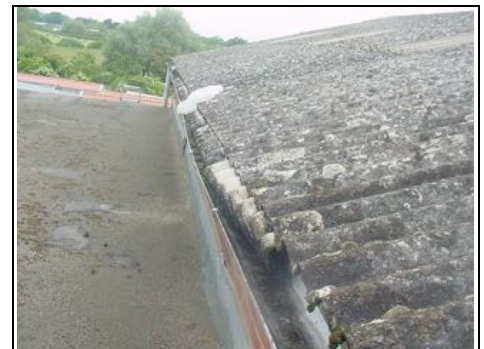
Asbestos roof
