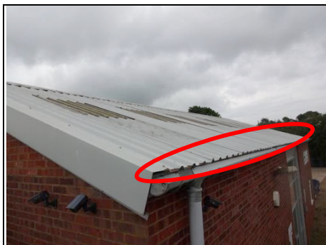
Edge/end of cladding is rusting
