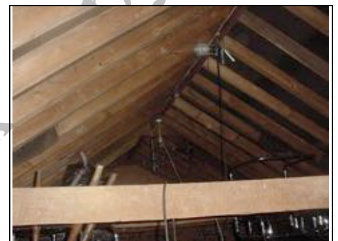
Main A Frame roof structure
