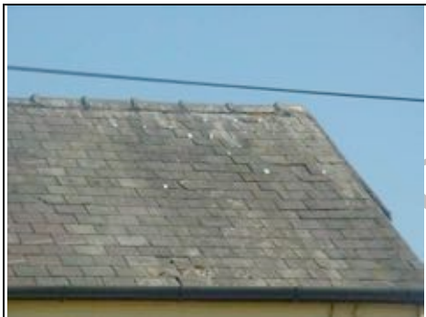
Slate lead tingles to the main roof
