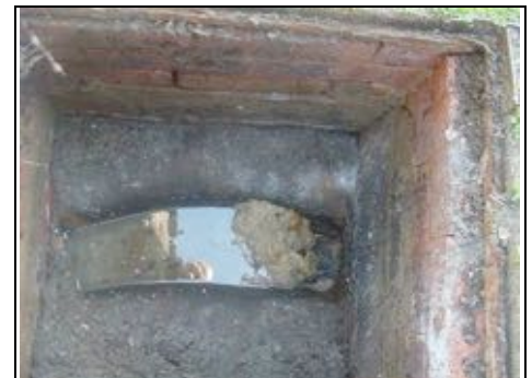
Blocked drain to the right of the property
