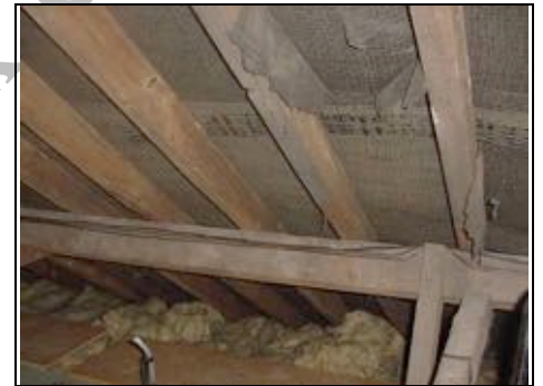
Hessian based felt
