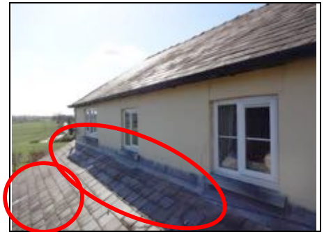
Slates repaired with lead tingles to the rear roof Ariel view – 360 photo
