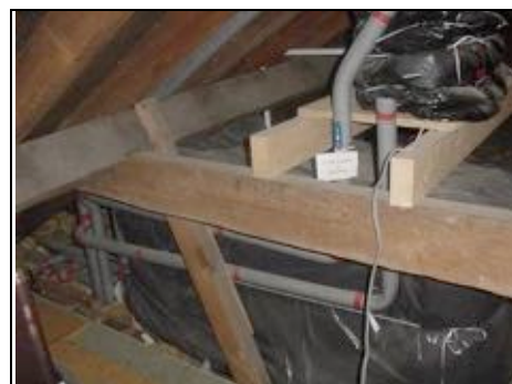
Water tank within the roof
