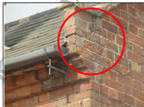
Hairline cracking and spalling brickwork to parapet wall to right side
