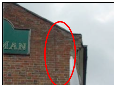
Cracking to parapet wall to left side
