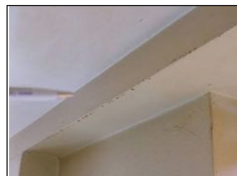
Grease dripping off kitchen ceiling
