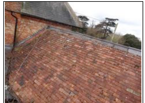
Deterioration to clay tile roof
