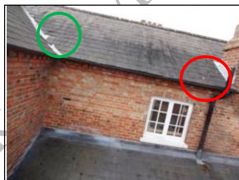
Slate roof to rear with displaced slates (green oval) and lead tingles (red oval) Aerial view – 360 photo
