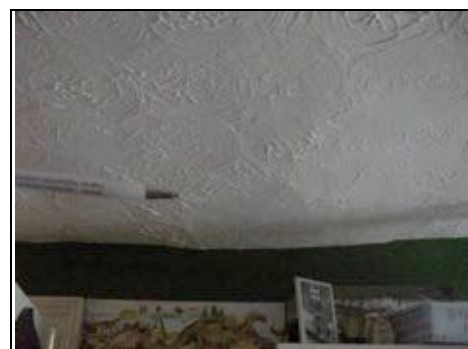
Undulations in rear right bedroom ceiling
