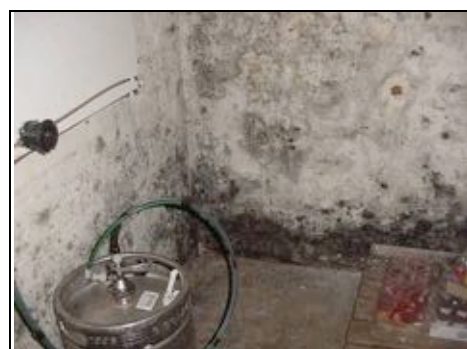
Dampness and black mould in cellar
