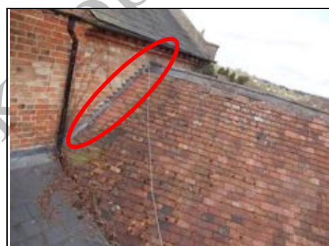
New tiles to clay tile barn roof Aerial view – 360 photo
