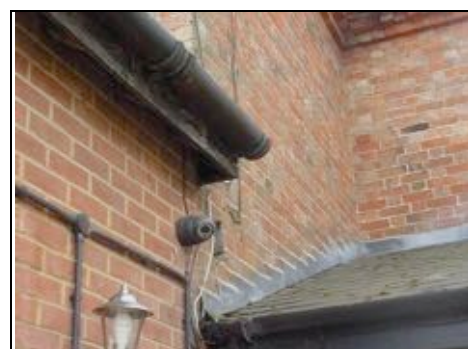
Parapet wall to left side cemented over
