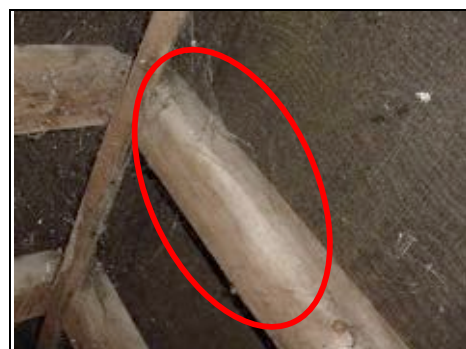
Signs of woodworm in roof over prep area
