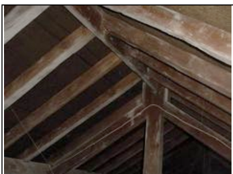
Condensation to timbers
