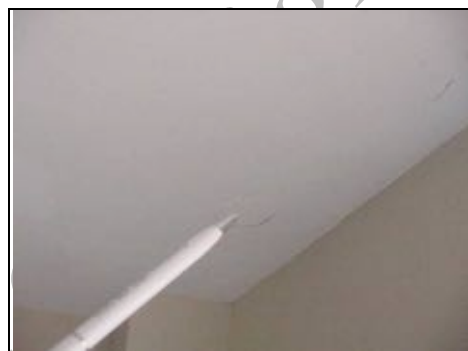
Damp staining from roof above
