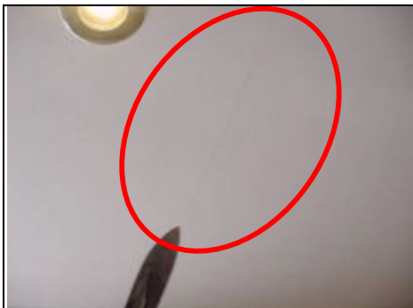
Hairline cracking to ceiling in gents toilets
