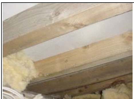
Modern breathable underlayer between timbers
