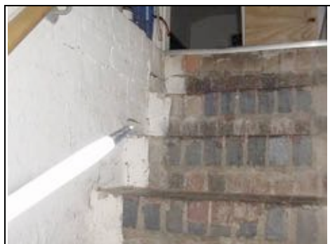
Crack in steps
