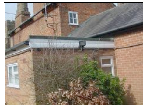
Low level pitched roof and low level flat roof over toilets
