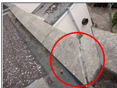
DIY repairs - mastic in the joints to the coping stone Aerial view – 360 photo
