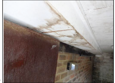
Box gutter leaking Aerial view – 360 photo
