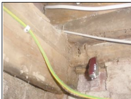
Knife into rotting timber
