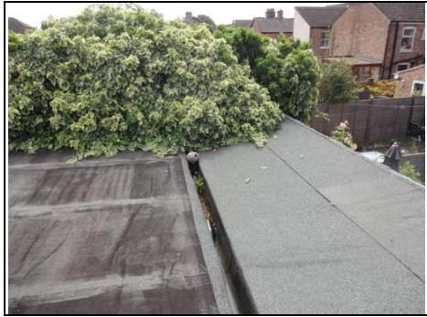
Rear left roof (no.8) and box gutter (with the ball at the end) Aerial view – 360 photo
