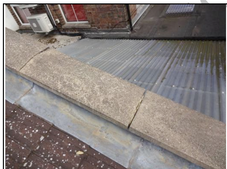
Weathering to coping stone joint Aerial view – 360 photo
