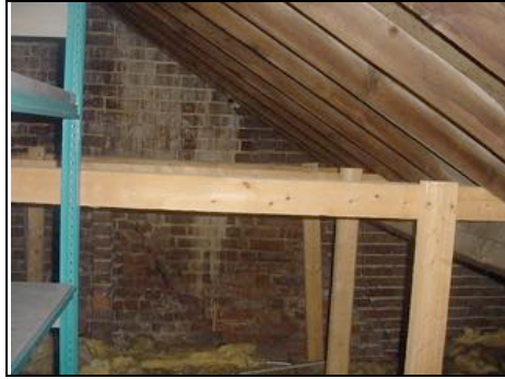
Constraint added likely to be roof spread
