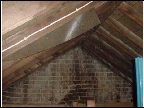
Main roof right side chimney dampness
