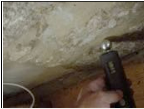
Testing for dampness in fireplace stonework
