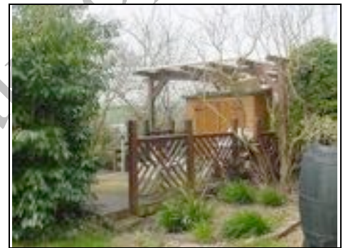
Septic tank area
