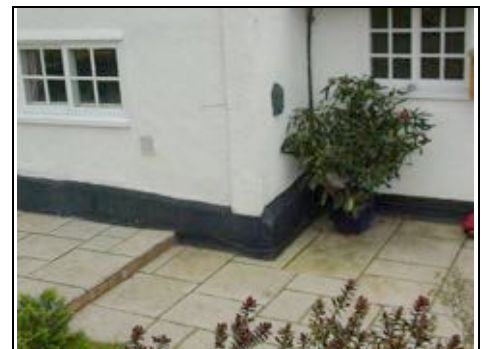
Paving around property
