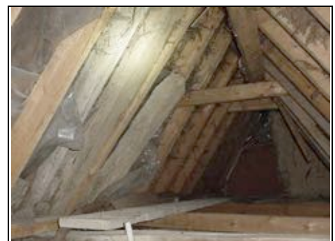
Mixture of new and older timbers to the centre roof
