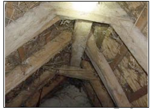
Timber to the right roof
