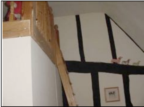
Wall structure showing the studs and infill panels
