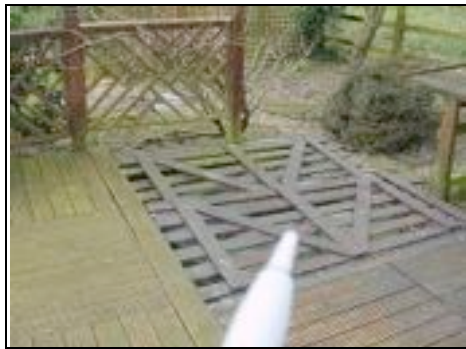
Top of septic tank
