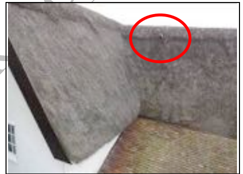
Flue ~ Aerial View - 360 Photo ~
