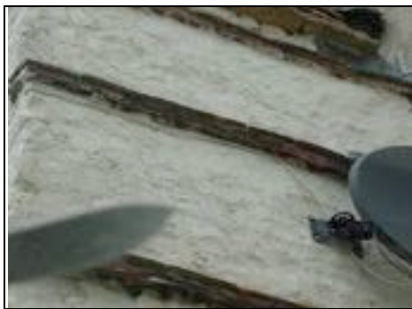
Cement repairs on stone chimney
