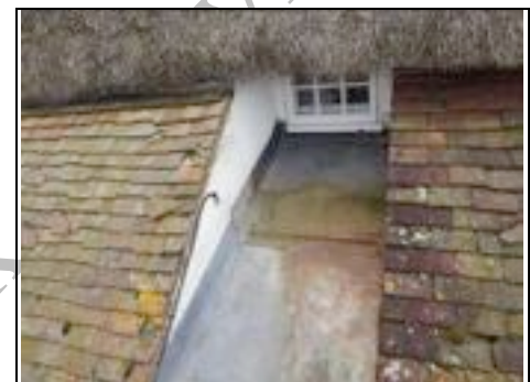
Lead valley to bathroom window ~ Aerial View - 360 Photo ~
