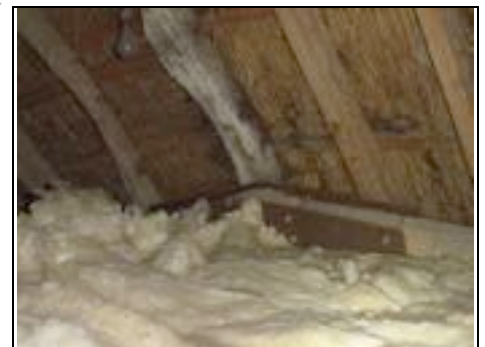
Brace at base of timber to left roof
