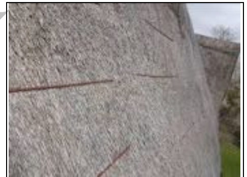
Stitch in time to thatch, rods added to hold thatch in place ~ Aerial View - 360 Photo ~
