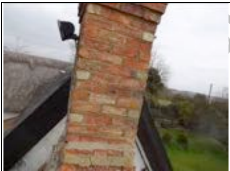
Close up of chimney
