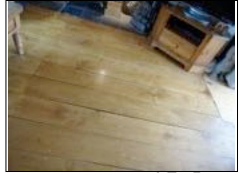
We were advised original floorboards were sanded and reshaped
