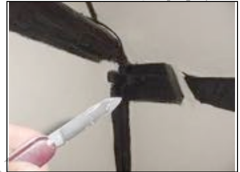
Brace added in middle wall on left side
