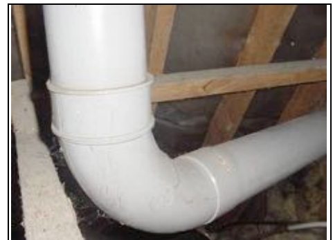
Plastic pipe within roof
