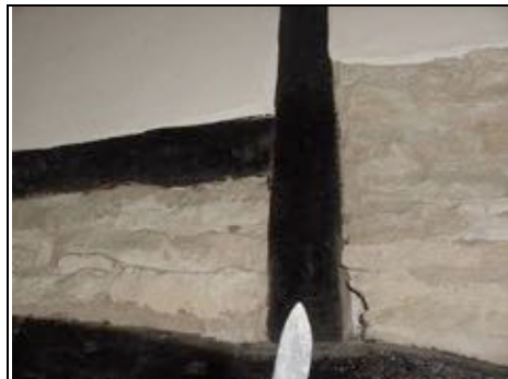
Infill panels and stonework
