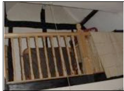
Mezzanine/roof access to right roof
