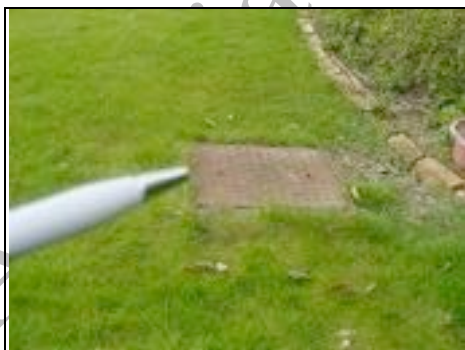
Manhole adjacent to garage
