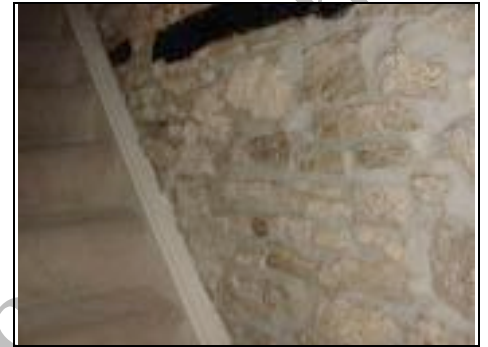
Cement repairs to stonework on side of staircase
