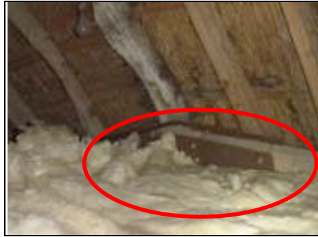
Brace at base of timber
