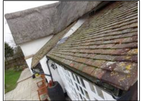
Gutters and downpipes to tiled roof
