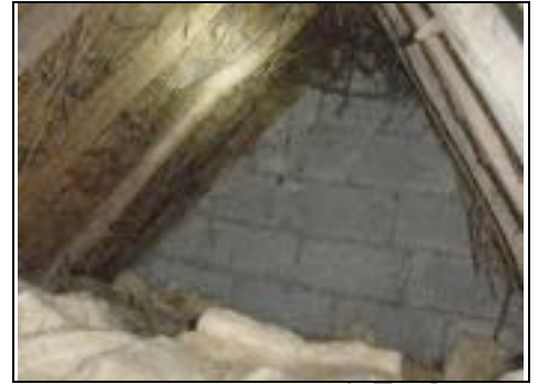
Stonework or blockwork?
