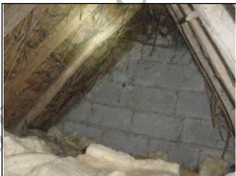
Stonework or blockwork?
