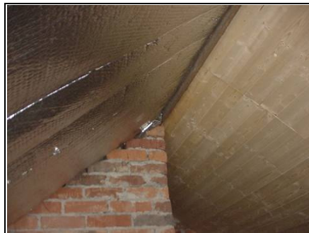
Foil insulation which has been put on at a later date
