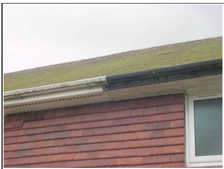
Vented soffit to left hand neighbour
