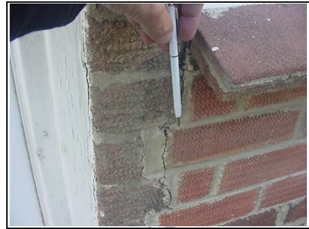
Pen indicating minor hairline cracking where some work has been carried out around the rear kitchen window
