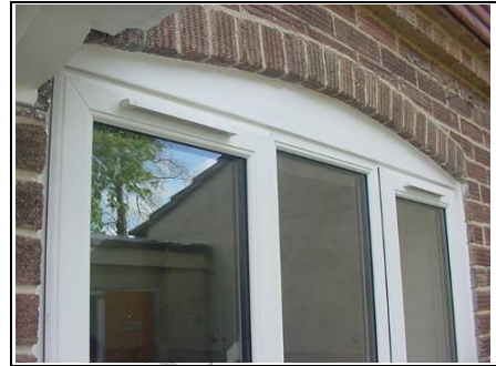
Plastic window with trickle vent
