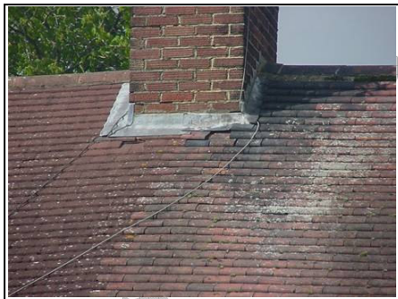
Undulation in the roof
