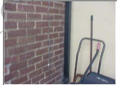
Stretcher bond brickwork
