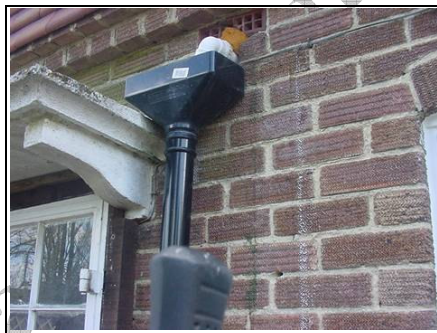
Overflowing hopper head
