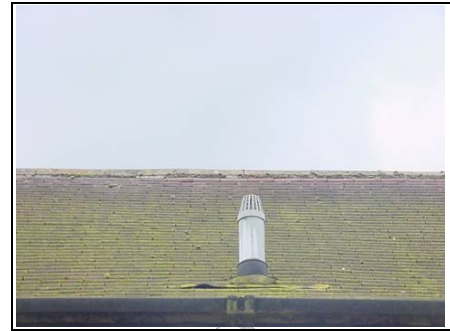
Soil and vent pipe
