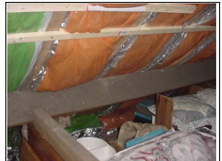
Bagged insulation that has been put on and securely battened at a later date
