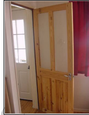
Wooden panel door with glazing
