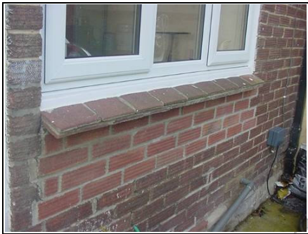
Brickwork amended under kitchen window
