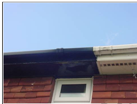
Vented soffit to right hand neighbour
