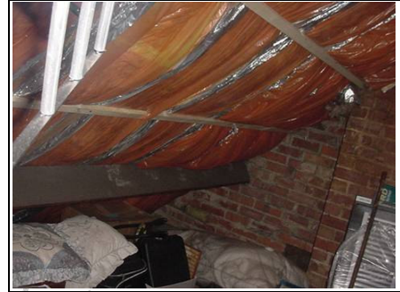
Insulation battened in place
