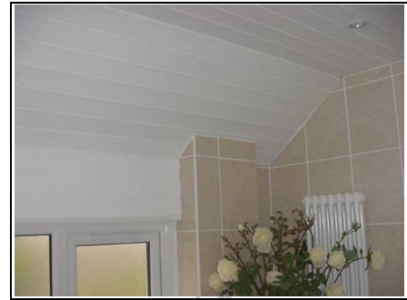
Cold bridging point where ceiling follows line of roof
