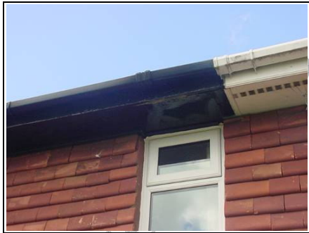
We can see some detonation to the fascias and soffits
