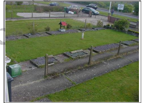
Concrete post and wire fence To right hand side area
