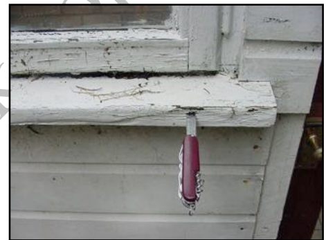
Timber window with rot
