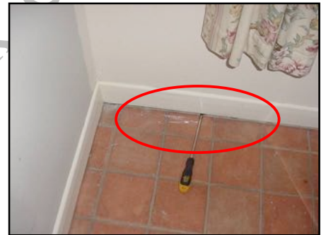
Gap between tiled floor and skirting board
