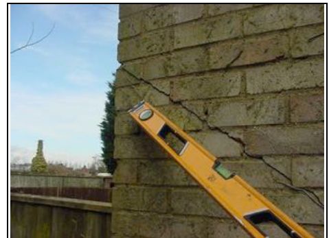
Cracking to garage wall
