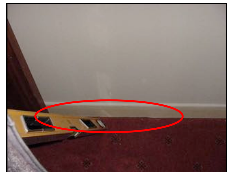
Gap between carpeted floor and skirting board
