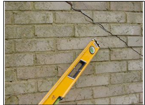
Cracking to garage wall
