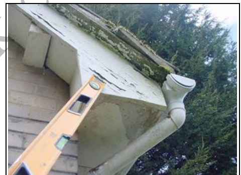
Deterioration to fascias and soffits
