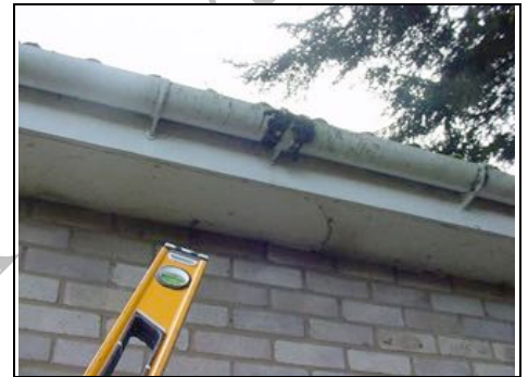
Leaking Gutter
