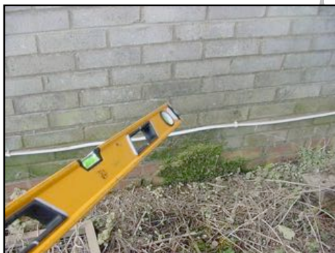
Gutter has leaked on to wall below
