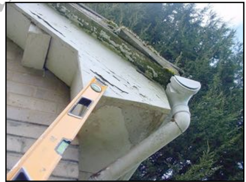
Fascias and Soffits in need of repair and redecoration
