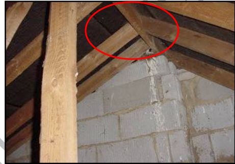
Roof structure - ridge board visible
