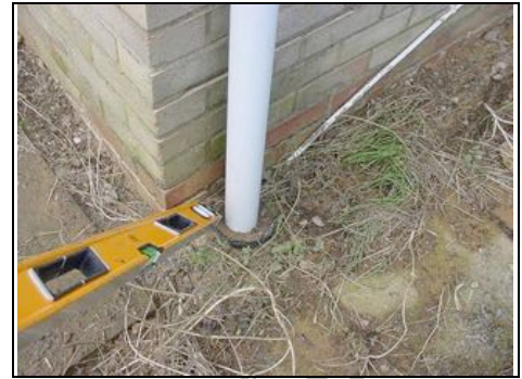
Downpipes feed directly into ground
