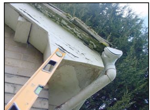
Deterioration to fascias and soffits
