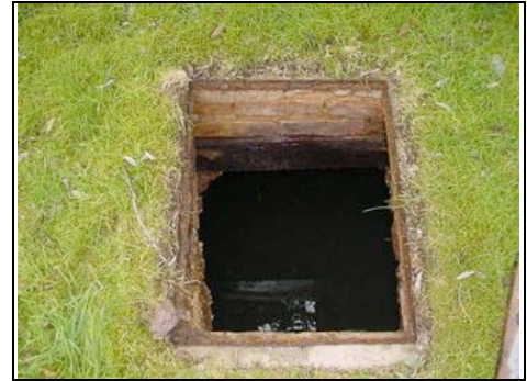
Manhole containing septic tank/cesspit
