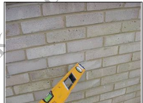
Stretcher bond brickwork
