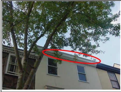
Georgian building with hidden box gutter
