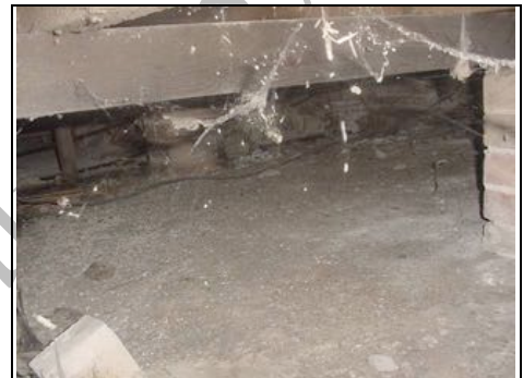
Looking to right side of property we can see brick piers and darker areas which indicate some dampness is getting in.
