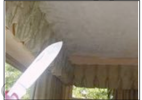
Dampness visible to lounge extension flat roof
