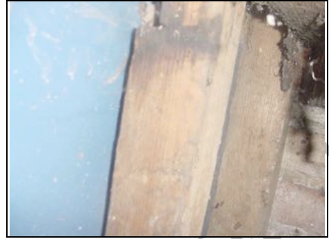
Timber supports around nearby chimney
