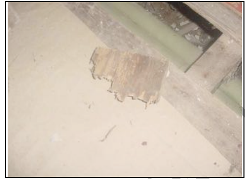
Loose piece of timber with woodworm found under floor
