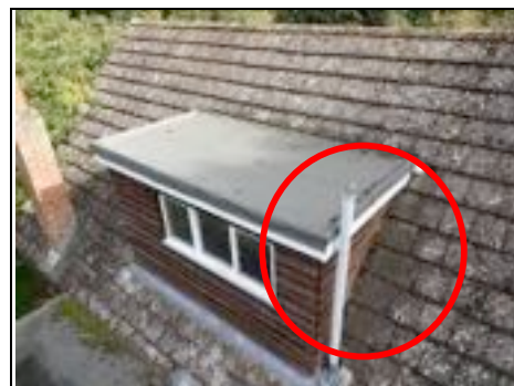
Soil and vent pipe
