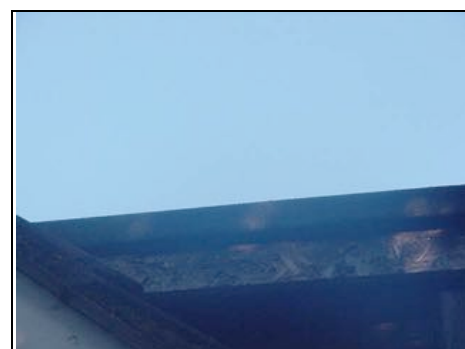
Fascia and soffit at high level replaced with sterling board
