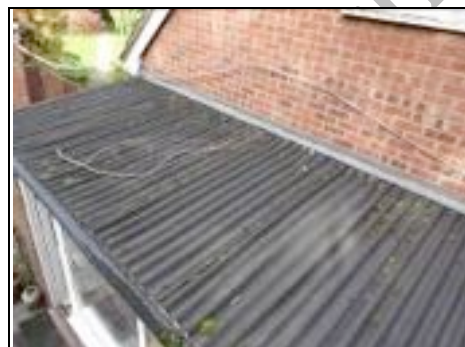
Possible asbestos roof
