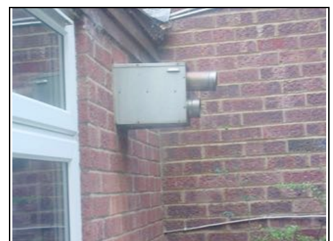
Flue from boiler
