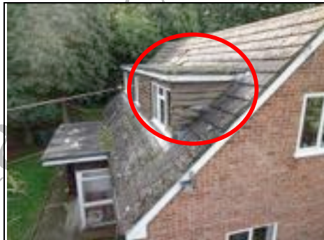
Flat roofs Timber cladding rotting and coming away on dormer
