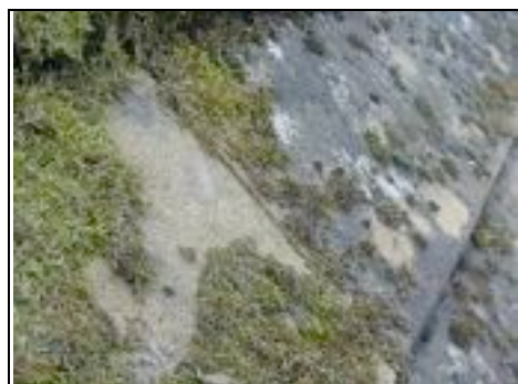
Moss to roof and marks where surface has deteriorated of tile
