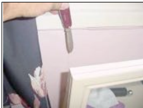
Hairline cracking right bedroom
