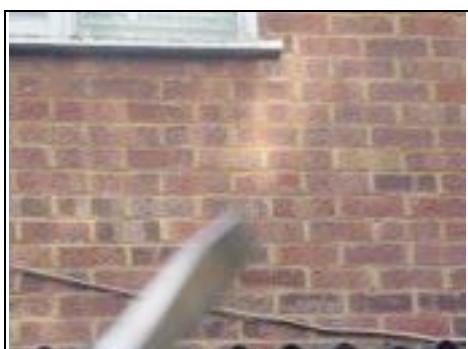
Crack in brickwork
