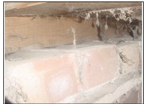
Detail where the floors sit onto the perimeter wall
