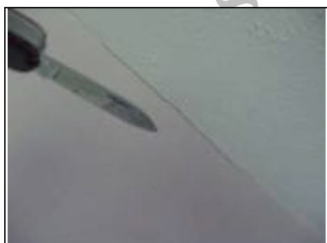
Hairline cracking right bedroom
