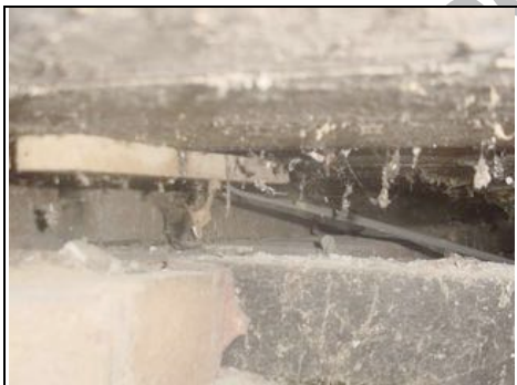
Cobwebs underneath floor indicating it is dry-ish. New piece of timber which are often added when floorboards are lifted for putting in central heating and wiring
