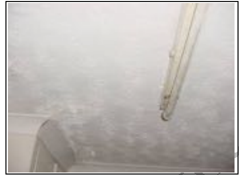
Condensation in ground floor bathroom
