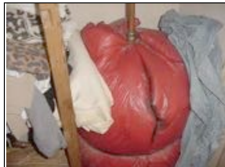
Older style hot water cylinder
