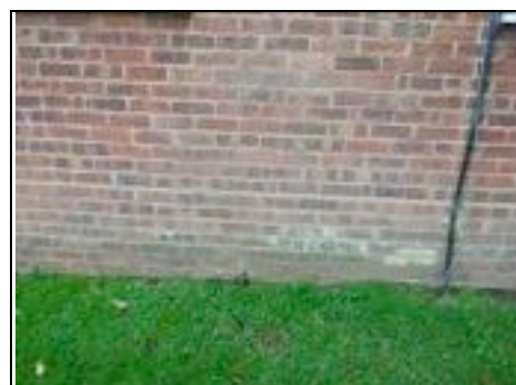
Stretcher bond brickwork
