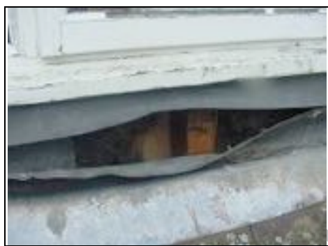
Exposed part at front of property shows timber frame
