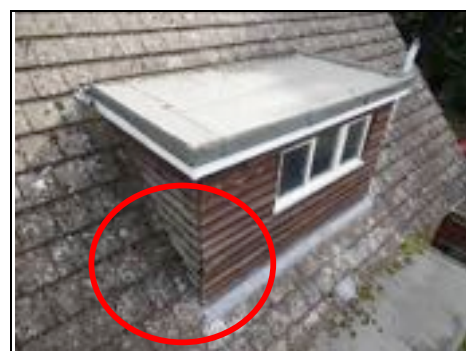
Deteriorating shiplap boarding to dormer
