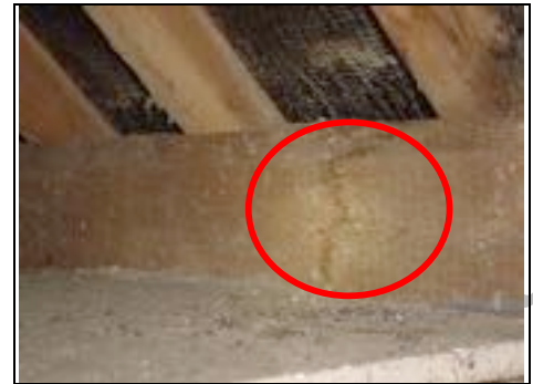
Staining coming through where pitched roof meets the flat roof
