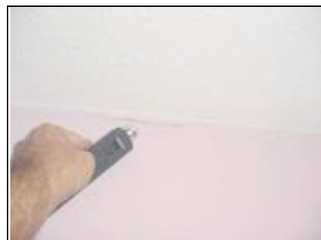
Cracking to high level in right bedroom
