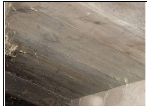
Underside of floorboards all looking in reasonable condition
