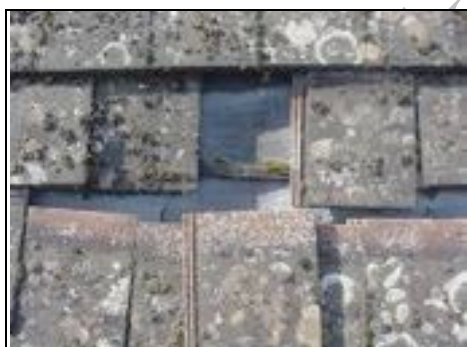
Roof tile missing
