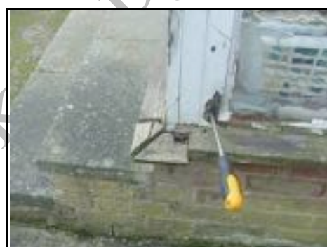
External joinery deteriorating
