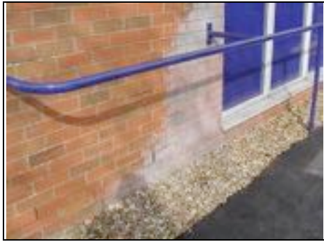
Staining to brickwork
