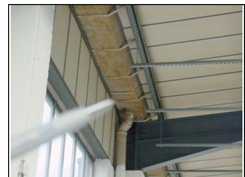
Water staining still visible
