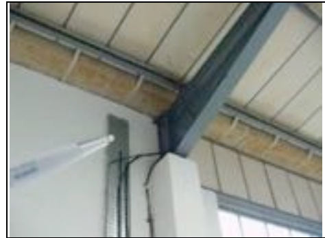
General lack of cleaning to the structural frame
