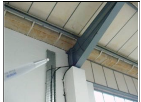
Structural frame not cleaned
