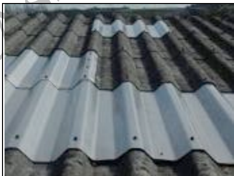
GRP overcladding of asbestos panels
