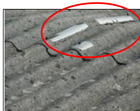
Old flashband repairs
