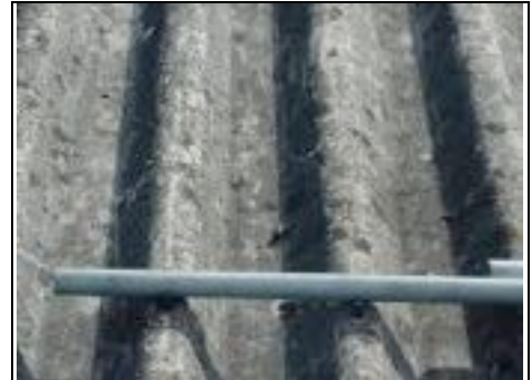
Close up of asbestos panel
