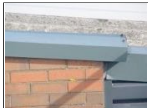
Upstand to the parapet wall
