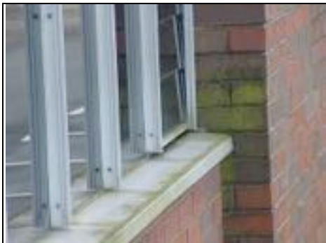
Green mould to brickwork and window staining
