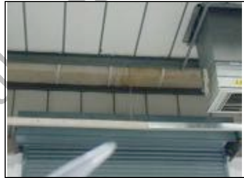
Staining and discoloration to the undercladding panels and underside of the gutter
