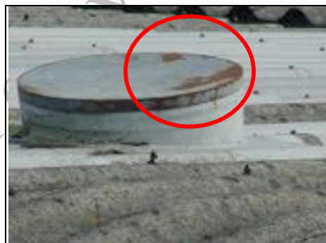
Rusting to top of the vent units
