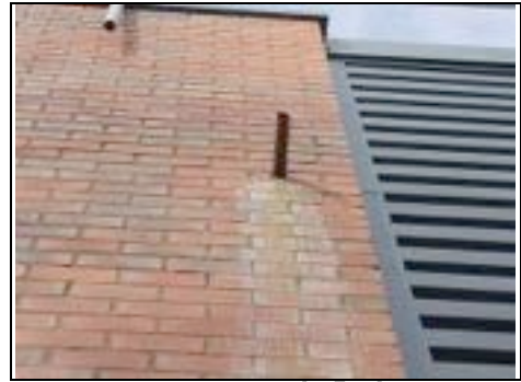
Staining to brickwork
