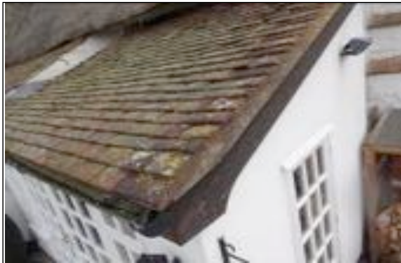
Spalling to tiles ~ Aerial View - 360 Photo ~
