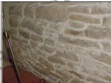
Dampness coming through and various repairs
