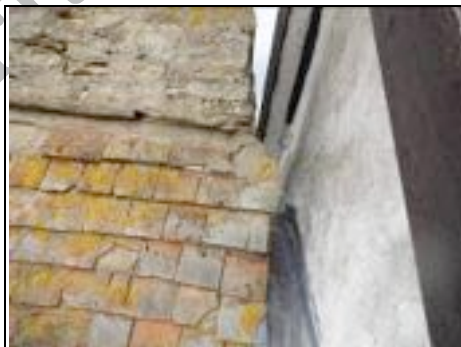
Gap between chimney and main building
