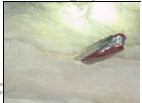
Knife going completely into timber common rafter
