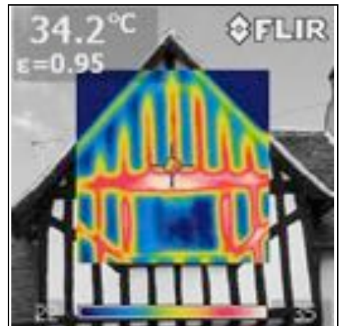
Thermal image showing heat loss around window of timber frame pub
