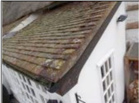
Spalling to tiles ~ Aerial View - 360 Photo ~
