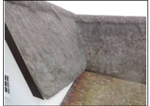
Thatch in poor condition
