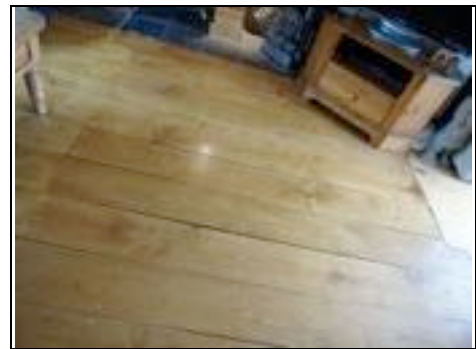
Replacement of original floorboards
