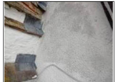
Mastic on lead to right gable
