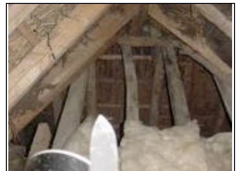
Deterioration/twisting to timbers in left roof
