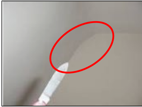
Hairline cracking in master bedroom
