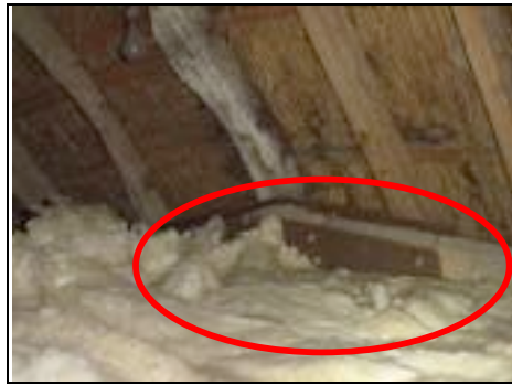
Brace at base of timber
