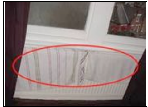
Drying washing on radiators can cause condensation
