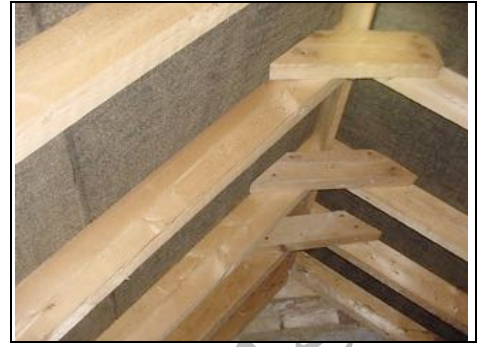
Roofing felt rather than protective underlayer
