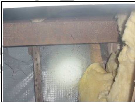
Plastic protective underlayer that causes roof to sweat/condensate
