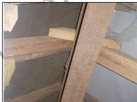
Rusting to RSJ in main roof
