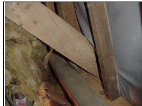
Nails coming through the plastic sheeting of protective underlayer
