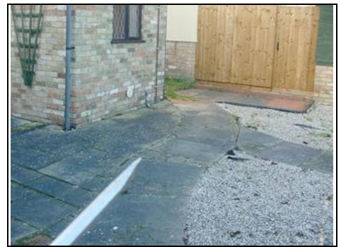
Movement in paving area
