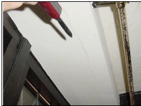
Cracking to middle reception room
