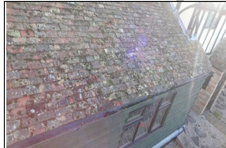
Tiles spalling and ending in gutters of single storey roof
