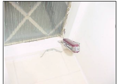
Wet rot to bathroom window
