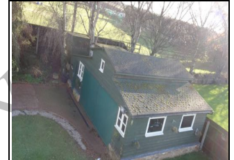
Shallow pitched mineral felt tile roof
