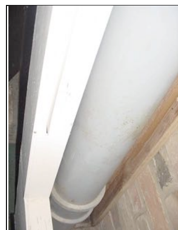
Soil and vent pipe going down within study
