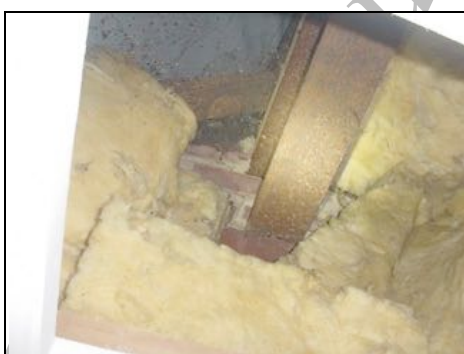
RSJ rusting in roof above bathroom
