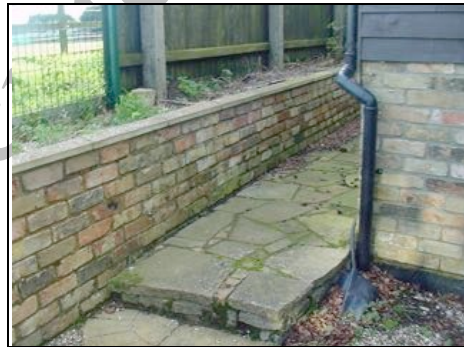
No weepholes to retaining wall
