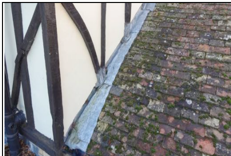
Leadwork to single pitched roof
