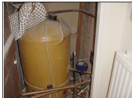
Factory lagged hot water cylinder
