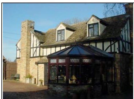
Front right chimney breast sits partly externally
