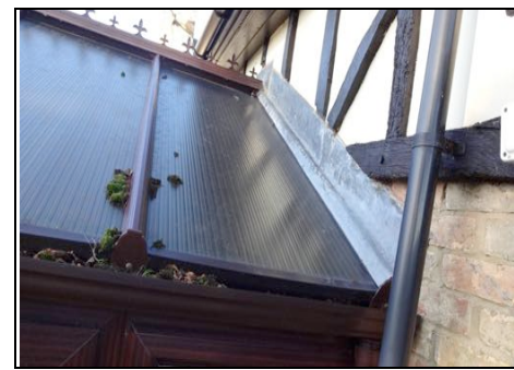
Moss is coming off main roof (right side) landing on the conservatory and then filling up the gutters
