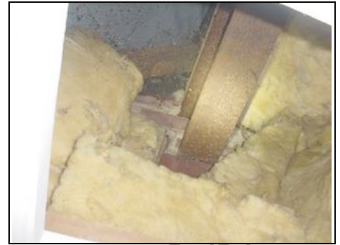
RSJ in roof above bathroom
