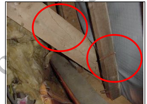
Split in timber in main roof Nails puncturing through the protective underlayer
