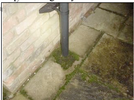
Downpipe feeding directly into ground with moss around it indicates that it gets blocked
