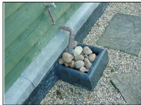
Lead detailing to the base
