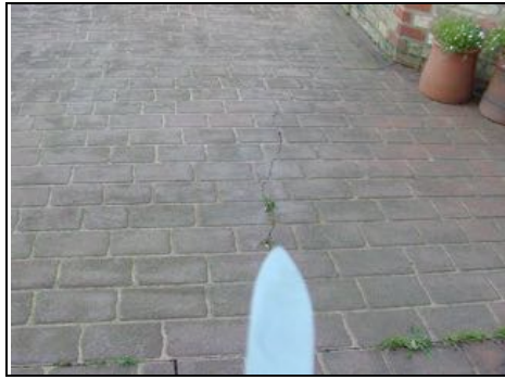
Crack in pressed concrete driveway
