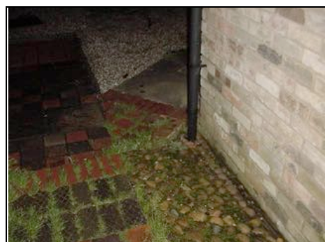
Downpipes discharging directly into ground
