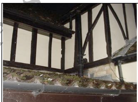
Plastic soil and vent pipe does not discharge high enough
