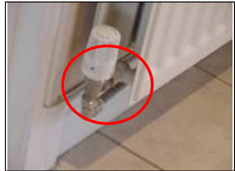
Mixture of plastic and copper pipes on radiator
