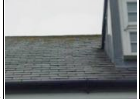
Undulation / lifting of slates which due to the height of the property and wind velocity could lead to lifting slates
