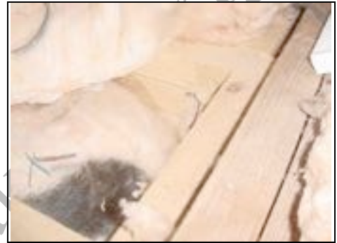
Backing to plasterboard
