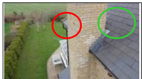
Left chimney with gutter positioned too close Aerial view – 360 photo
