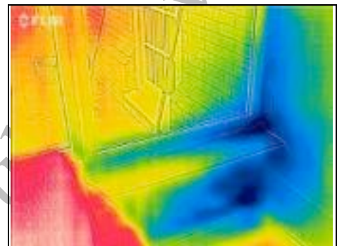
Conservatory, where meets main building on the right side corner (all directions given as you face the property). We can see the coldness/dampness
