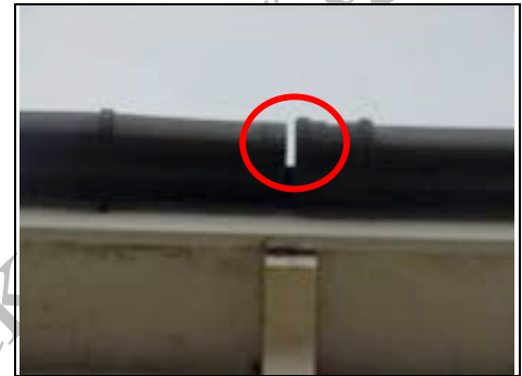
Gap in gutter to front
