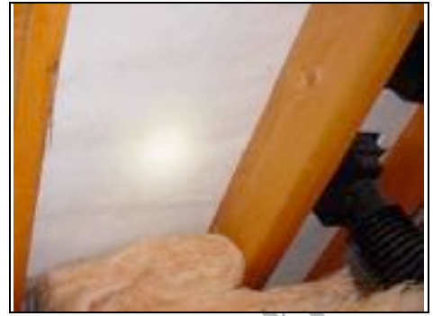
This photo shows the common rafters (the ones that form the pitch of the roof) and the white area between is the underlayer
