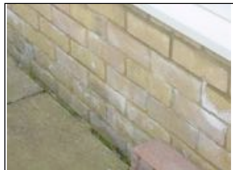
Efflorescence to base of conservatory
