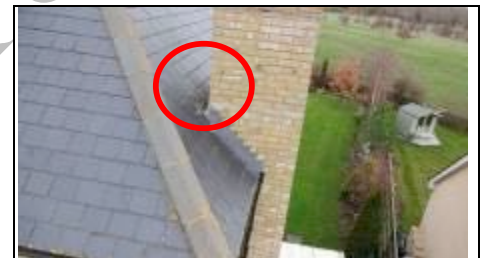
Trap behind chimney where dampness tends to get in
