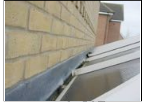
Close up of awkward valley between conservatory and main building
