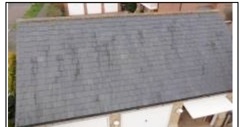
Garage roof where slates are missing
