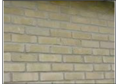
Some areas of repointing to brickwork
