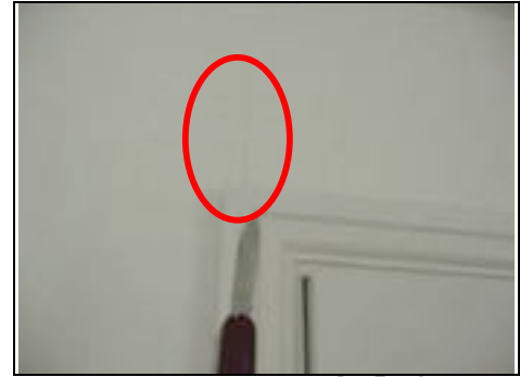
Hairline crack around one of the doors
