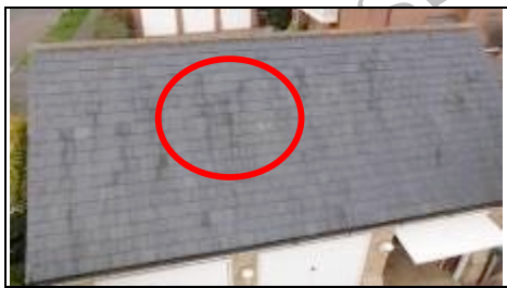
Missing slates to front Aerial view – 360 photo
