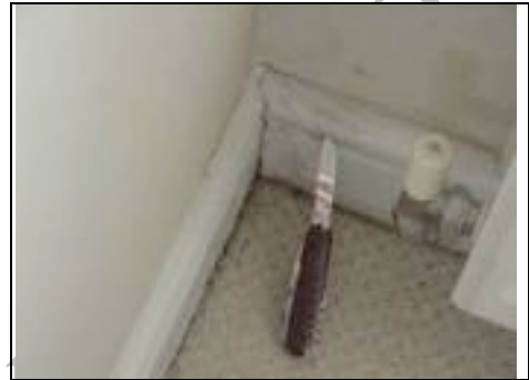
Dampness internally to skirting next to front right dormer
