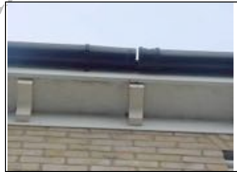
Rafter feet Also note gap in gutter
