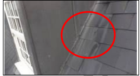
Problem with slates around front right dormer Aerial view – 360 photo
