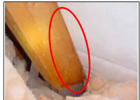
Damp staining to timbers
