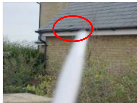
Missing slates to rear
