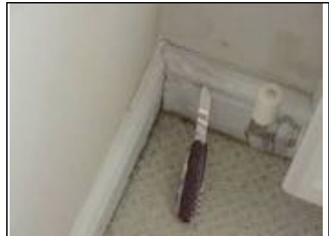
Dampness to skirting to base of front right dormer
