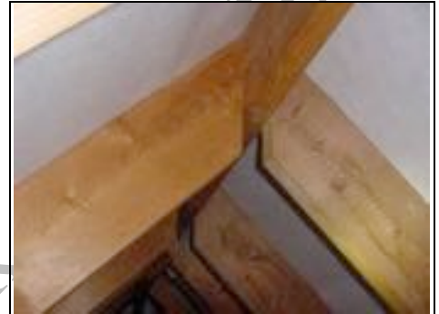
Unusual ridge board – partially pre-fabricated
