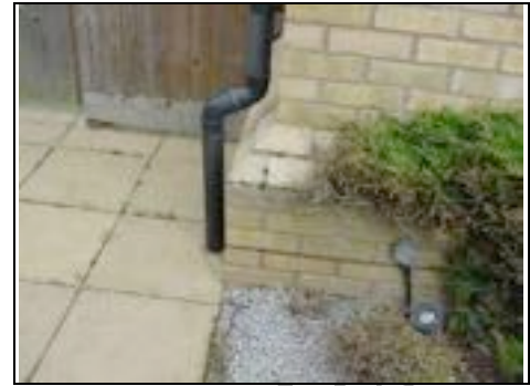
Downpipes feed directly into ground
