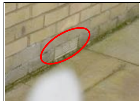
Airbrick acting as a gutter to conservatory
