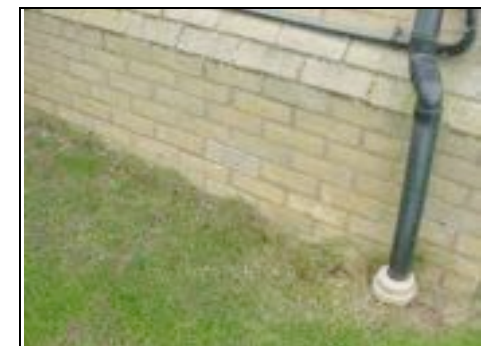
Downpipe going directly into the ground
