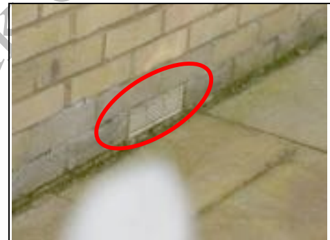
Airbrick acting as a gutter to conservatory
