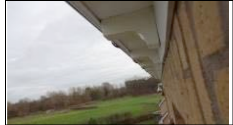
Plastic fascias and soffits with rafter feet
