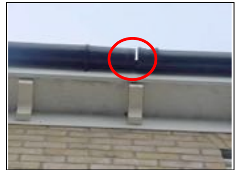
Gap in guttering to front
