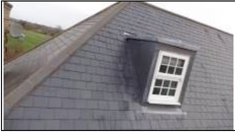
Very slight lift in slates to left side of front left dormer
