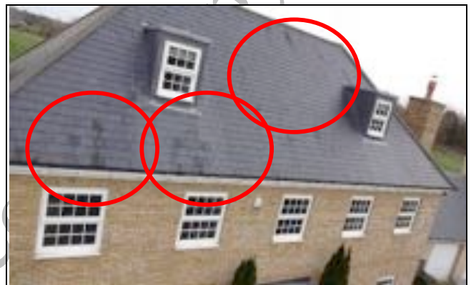
Darker deteriorating slates?
