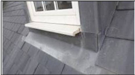
Close up of front right dormer where dampness is coming in Aerial view – 360 photo
