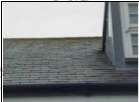
Undulation / lifting of slates which due to the height of the property and wind velocity could lead to lifting slates
