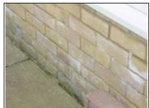
Efflorescence to base of conservatory
