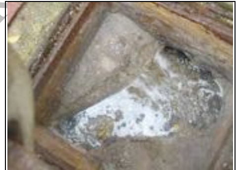
Drain blocked. Looks DIY as haunchings not formed properly.
