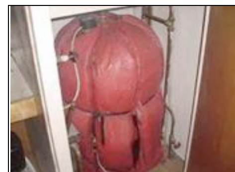
Older style cylinder with loose insulation jacket
