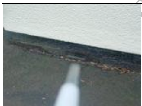
Airbrick to front acting as gutter
