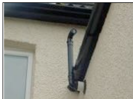
Flue from boiler on rear wall
