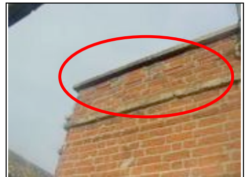
Chimney closed up and vented
