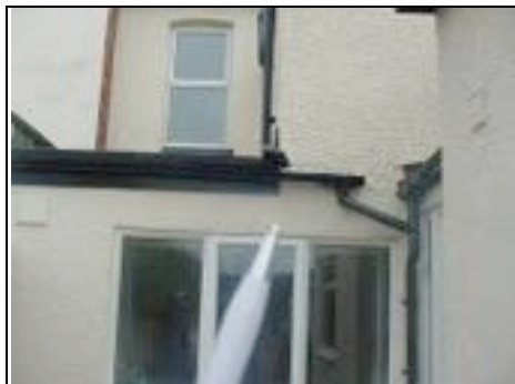
Beam supporting outside wall
