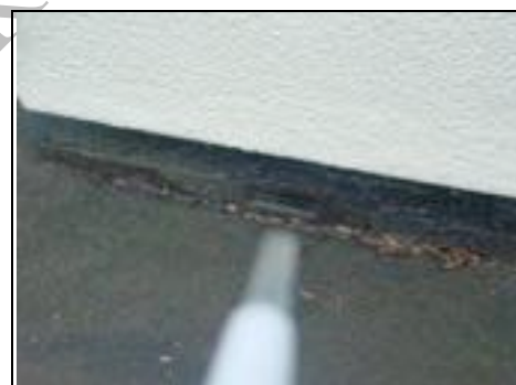
Airbrick to front acting as gutter
