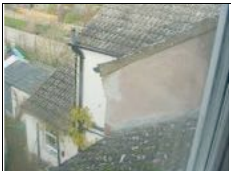
Inside plaster/render used outside
