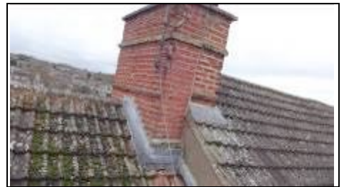
Chimney wrongly repointed in cement mortar
