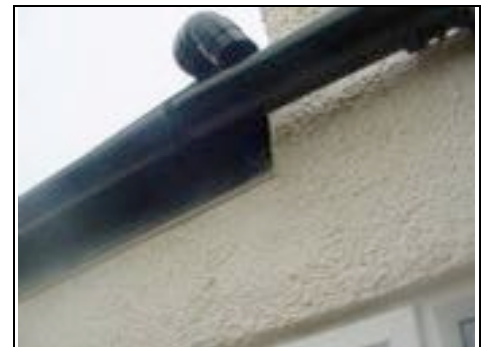
Gutters likely to overflow to kitchen
