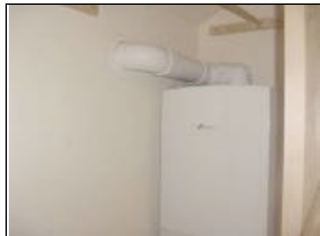
Boiler needs to be vented to outside air
