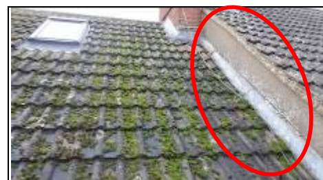
Cement mortar come away from flashing
