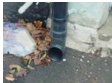
Downpipes discharge directly onto ground
