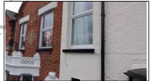
Cement based roughcast render to your property, Flemish bond brickwork next door
