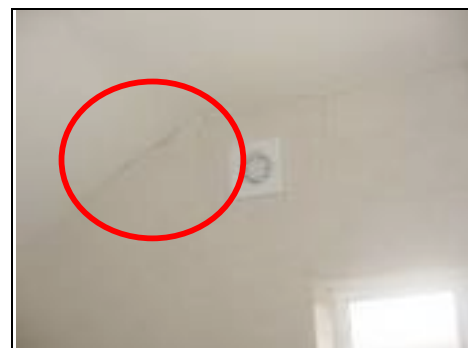
Small extract fan in bathroom Is this black mould (circled)? Conditions ripe for black mould
