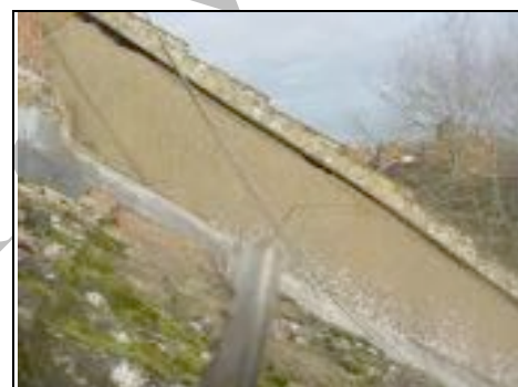
Cracking to render, flashing come away above rear blue bedroom where plaster has lost its key
