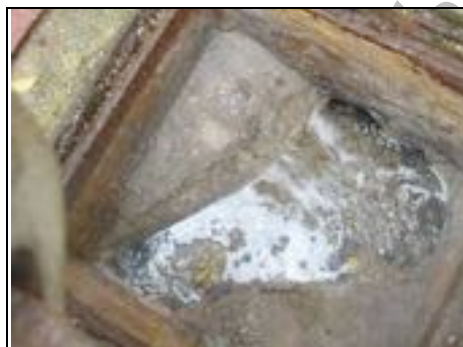
Drain blocked. Looks DIY as haunchings not formed properly.
