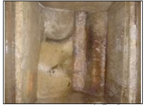
Example of manhole with haunching done properly
