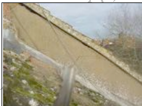
Cracking to render, flashing come away
