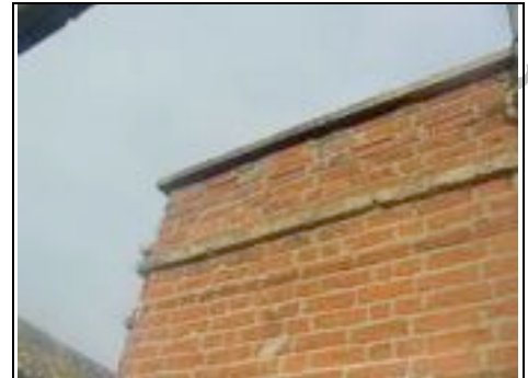
Chimney closed up and vented
