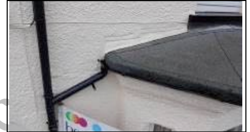
Guttering and downpipe from bay window roof, this could overflow and leak onto the wall causing dampness
