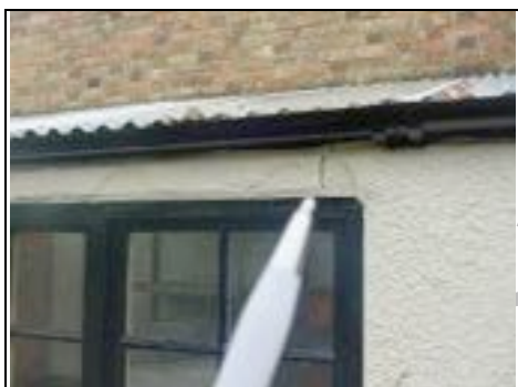
Crack in outbuilding
