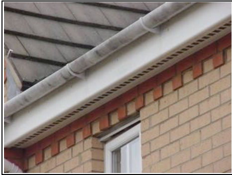
Ventilation in soffit boards
