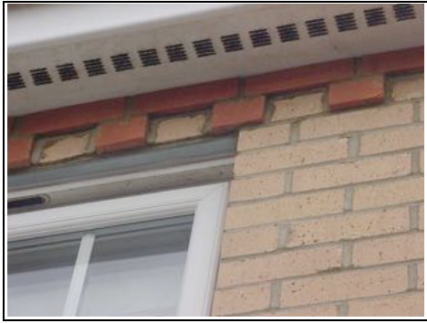
Corbelling below soffit
