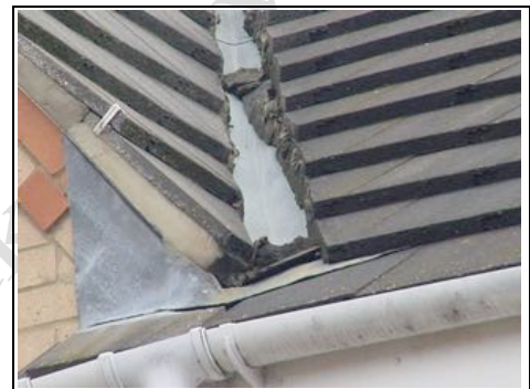
Cement mortar has come away
