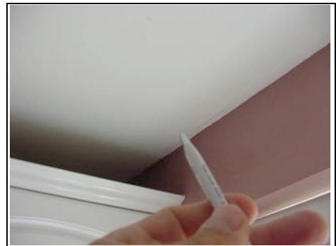
Hairline cracking to ceiling
