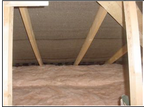
Mass of insulation in roof space
