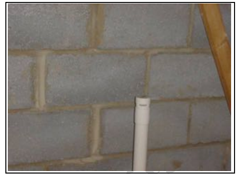
Air inlet valve trade name of Durgo valve
