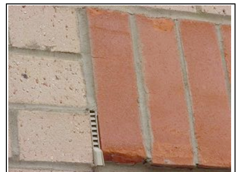
Spalling to red brickwork
