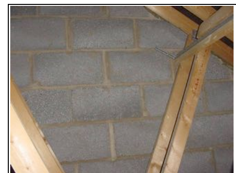
Blockwork firewall
