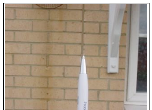
Mastic joint between two buildings
