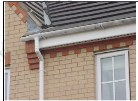
Gutter and downpipe
