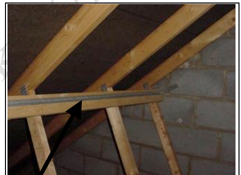
Strap that ties pre-fabricated trusses together
