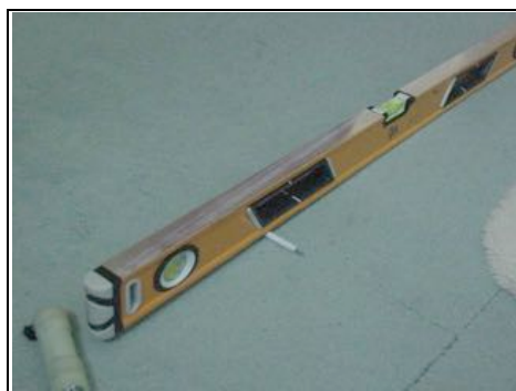
Dip in bathroom floor
