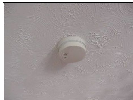
Hard wired smoke alarm
