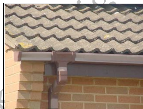
Old style plastic guttering affected by sunlight
