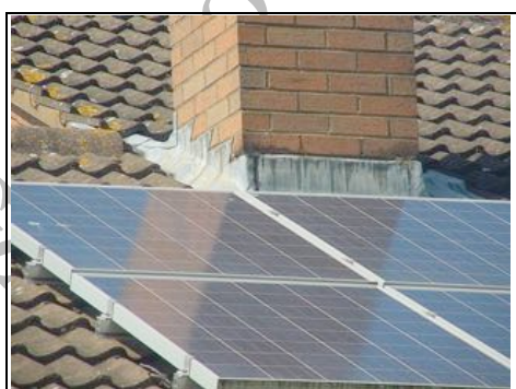
Left chimney - lead flashing and pointing needs checking
