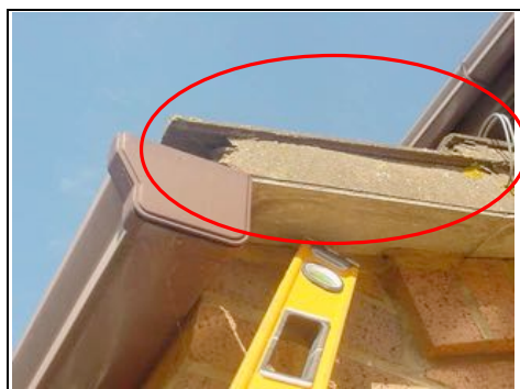
Asbestos roof verge
