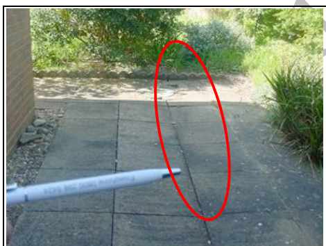
Dip in ground - drains right hand side following the drainage run
