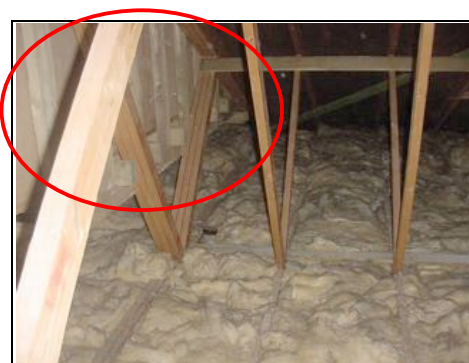
Boxing around the roof window in loft area
