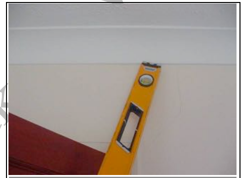
Crack above door in bedroom – rear left
