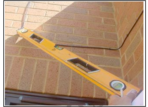
Step crack to rear of property
