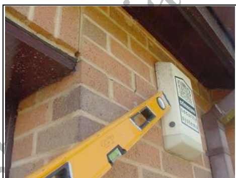
Step crack to right hand side
