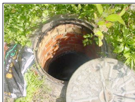
Brick manhole- front right
