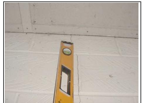
Cracking right hand wall
