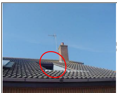
Roof window and lead surround area /detailing
