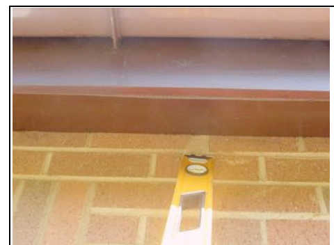
Slightly wide joint in pointing in some areas
