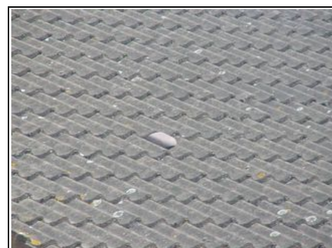
Vents in the roof
