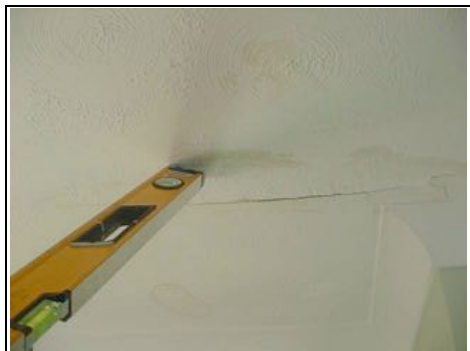
Staining and crack in reception room, from leak in chimney
